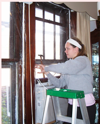
A volunteer from Villa Duchesne High School weatherizing a client's home.
