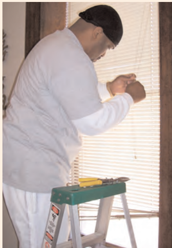
EnergyCare staff member weatherizing a window in a client's home.
